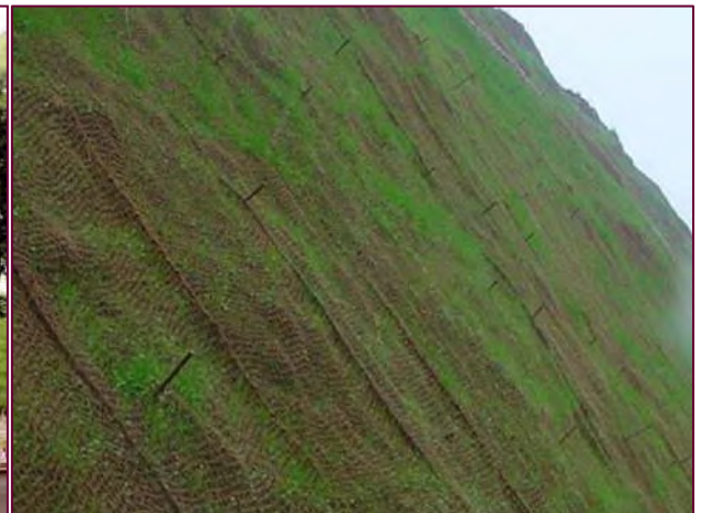
Coir Geotextile with Vetiver grass for stabilizing steep slopes
