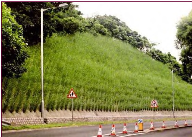
Coir Geotextile with Vetiver grass for stabilizing steep slopes
