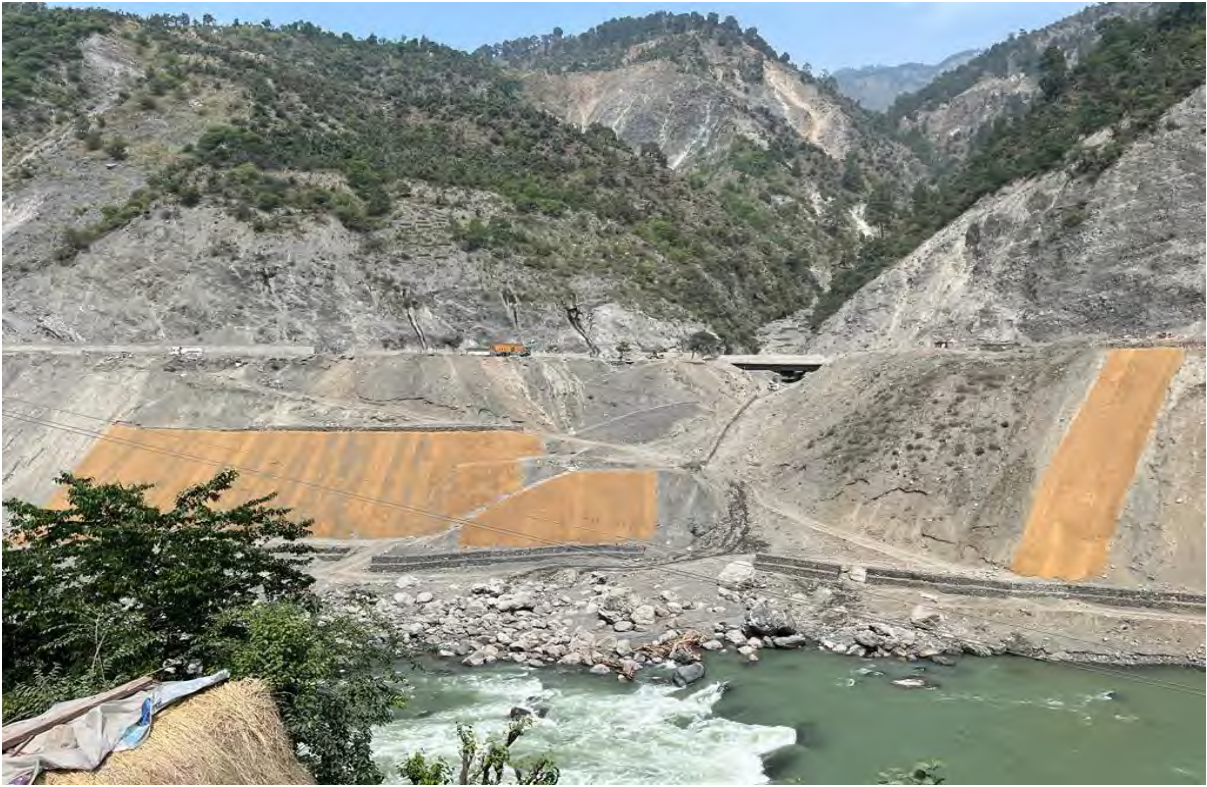
Dumping Yard at Karol Km 143+200
