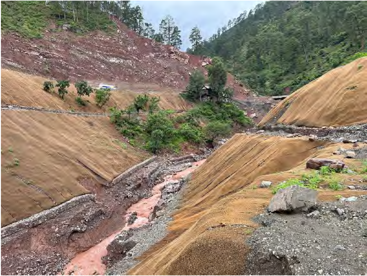
Dumping Yard at Peerah Km 135+600
