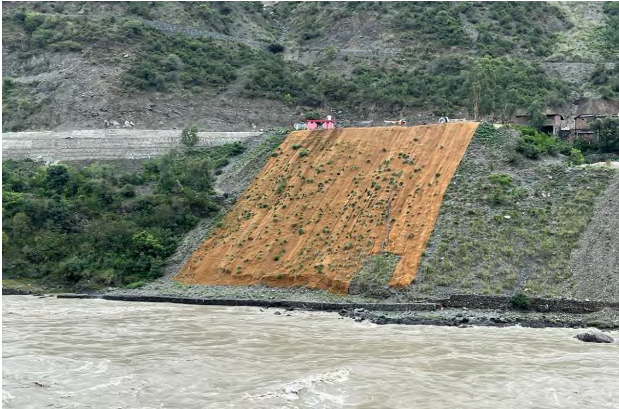
Dumping Yard at Mehar Km 145+570
