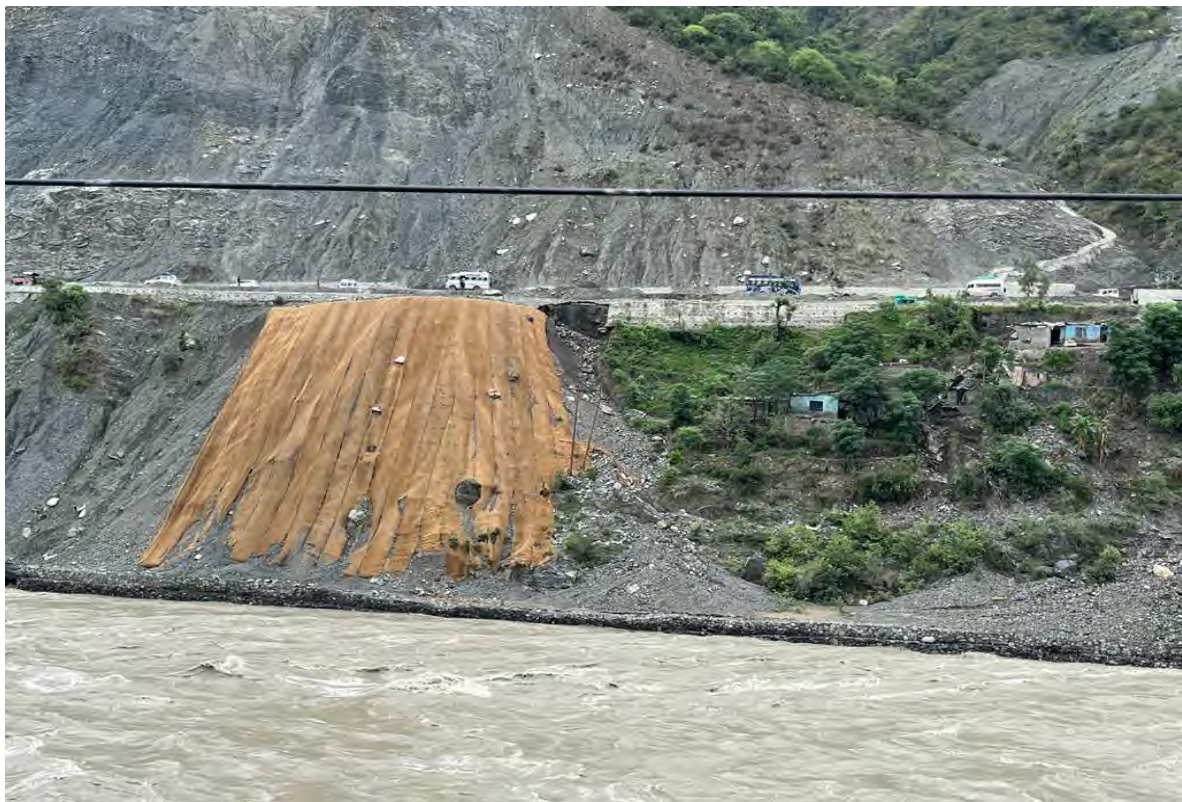
Dumping Yard at Mehar Km 145+470
