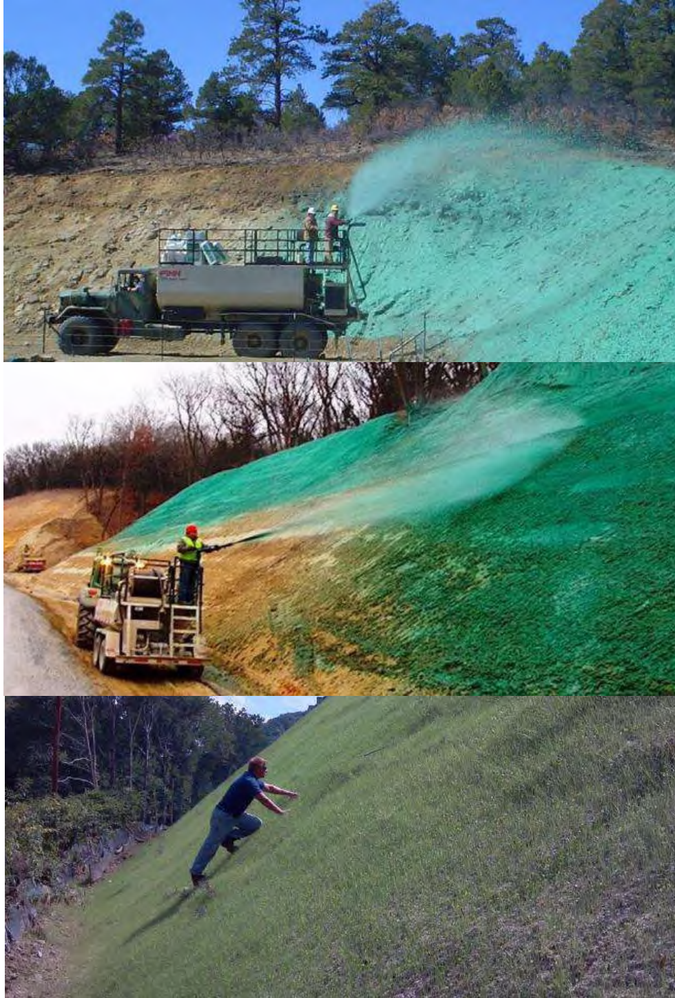
Hydro-seeding is ideal for steep slope
