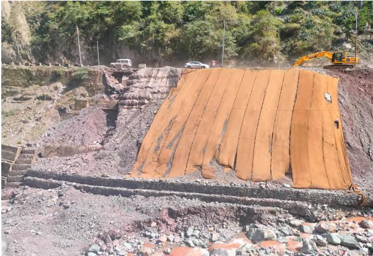
Dumping Yard at Kunfer Km 139+200
