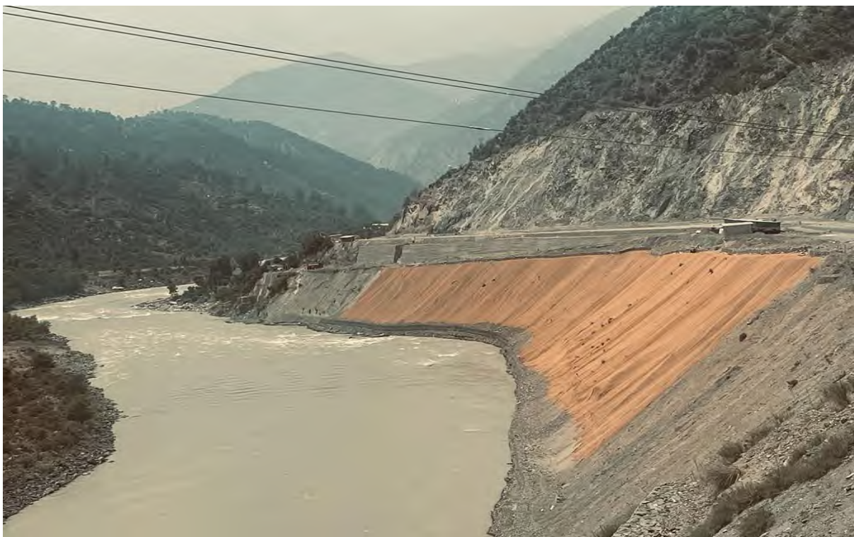
Dumping Yard at Trishul Morh Km 151+00
